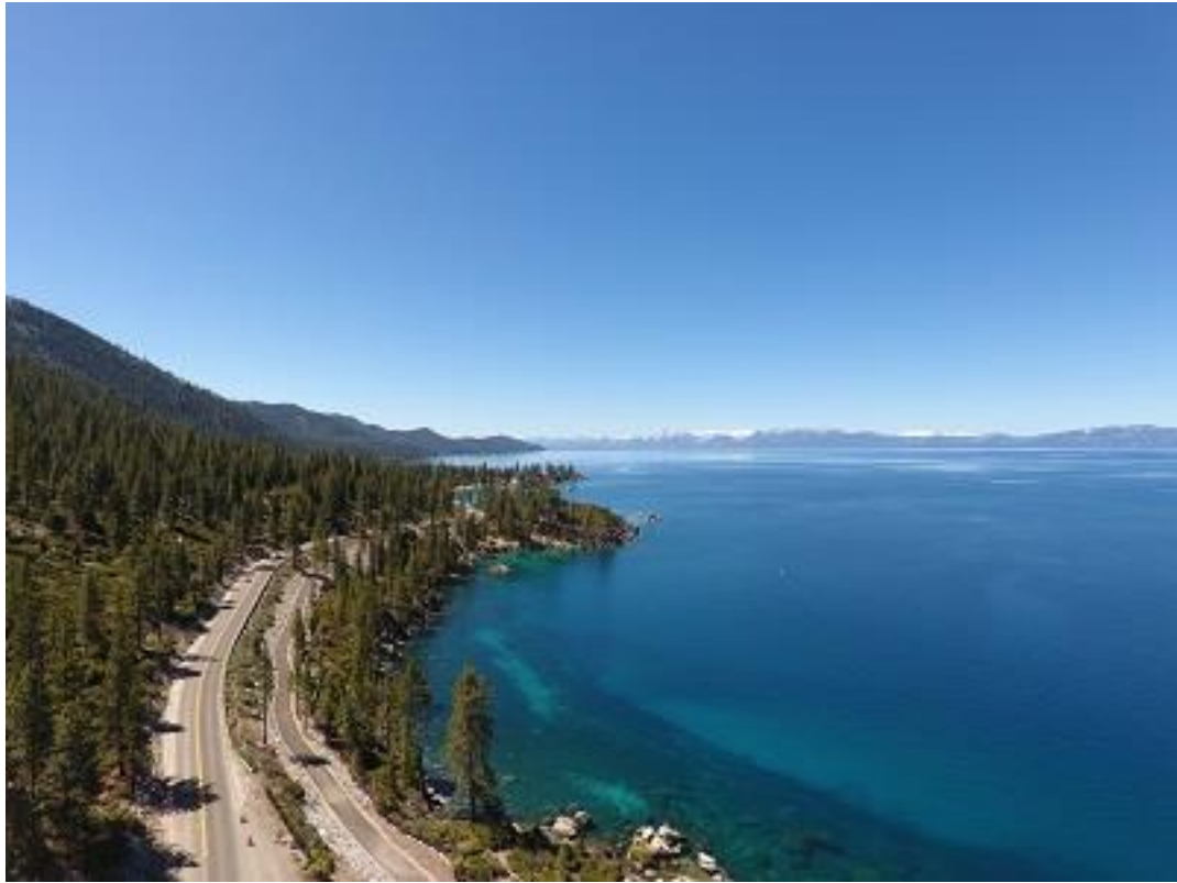
Construction work on State Route 28 shared-used path from the southern end of Incline Village to three miles south of Sand Harbor State Park will be on hold during the holiday week, July 2-6. Photo taken June 1, 2018 Courtesy: Granite Construction.
